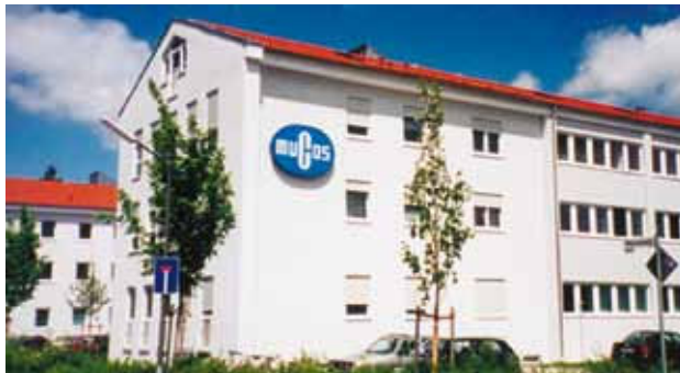
Company HQ in Geretsried
